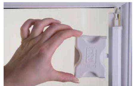
9. Fit the side profile retaining clips supplied. Always fit top clips approximately 100mm below top bracket. On longer drops fit additional clips evenly apart.
