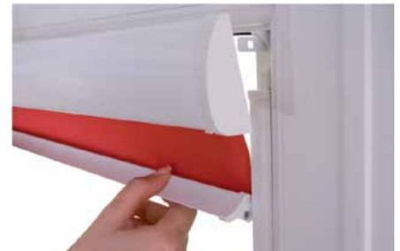
12. There are two methods of inserting the bottom bar/fabric into the side profiles. Method 1 (as above) is to slide the bottom bar and fabric into the side channels prior to attaching the fascia assembly (next operation).
