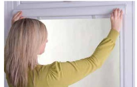
18. Ensuring the fabric is located within the side profile channel, press upwards on the finger release lever and push the fascia fully home. (Should removal of the fascia be desired reverse all processes and simply press upwards on the finger release levers to pull the fascia assembly away from the window).
