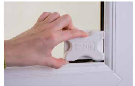
6. Insert the bracket behind the rubber seal until the tool edge touches the bead at both bottom & side. Repeat for other side.
