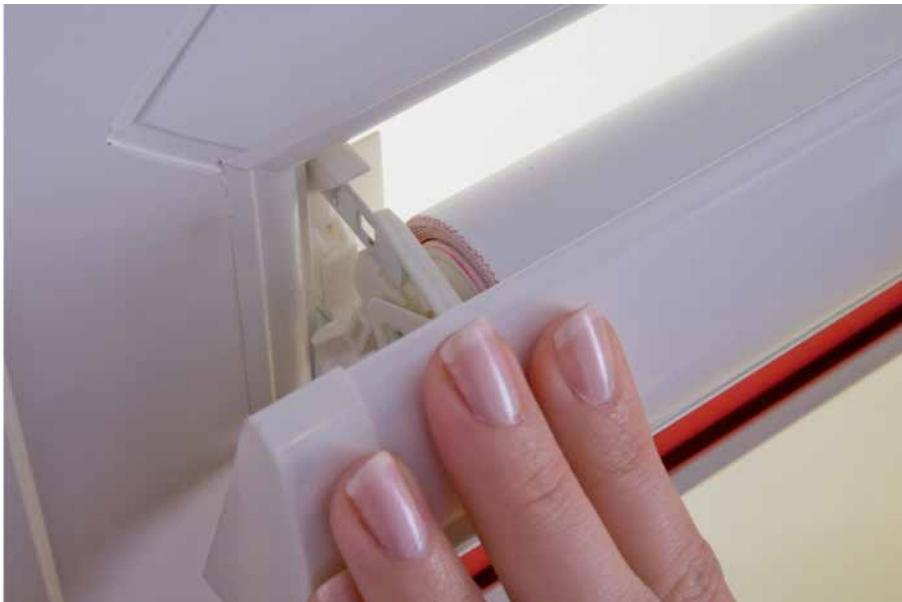
13. Carefully position the assembly and locate the fascia brackets over the top window brackets. Only push fascia half way home.
