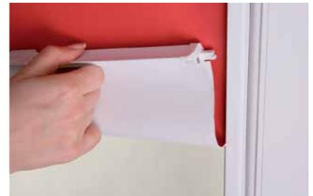
14. In method 2 attach fascia assembly as in step 13. Insert the fabric by carefully tilting up the bottom bar and fabric; locate the lower end into the side profile and then insert the upper end into the opposite profile channel.
